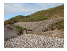
The visible sections of the main Seaham sea wall and promenade are in fair condition (below left), with most construction joints adequately sealed, but some minor gaps starting to become apparent at occasional joints. There are cracks at the joints between all three sets of access steps and their intersections with the main wall (below right), but there is relatively little abrasion damage and no obvious signs of cracking or settlement along the main wall itself.
