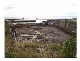
Along South Dock, considerable dock-related activity was ongoing (below left) so the structures at the root of the South Pier were only inspected from a distance. Rubble has been tipped along the seaward face of South Pier in one area fronting South Dock, with rock revetment then continuing to provide a more formal defence further south (below left).
