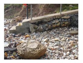
A local slope failure has occurred within Crimdon Park Caravan Site. Approximately 100m north of the Crimdon Park access steps, the timber fencing has been lost over a length of approximately 10m. A temporary barrier has been erected from steel tubing and plastic fencing with warning signs erected to warn members of the public (below).
