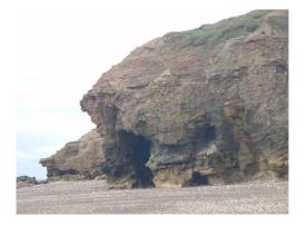
Gin Cave is an extensive cave with multiple openings (below left). The cave roof and walls appear relatively stable although there is evidence of historic failure as a large piece of rock has fallen from the roof above the northern entrance and now stands on the foreshore (below right).
