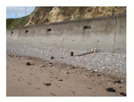
The beach levels at the time of the inspection were high, with a cobble berm overlaying the sandy foreshore and covering parts of the face of the wall to varying levels along the frontage (below left). This meant that the lower sections and toe of the sea wall could not visually be inspected. At the southern end of the frontage, towards Featherbed Rocks, the beach levels were highest and in one place shingle and cobble is blocking the drainage holes in the crest wall (below right).
