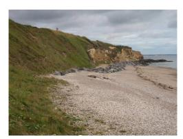
Along the lightly defended or undefended cliffs south of the formal revetment, there is evidence of ongoing slumping in the cliffs (below left), revealing soil netting in places near the access steps (below right).
